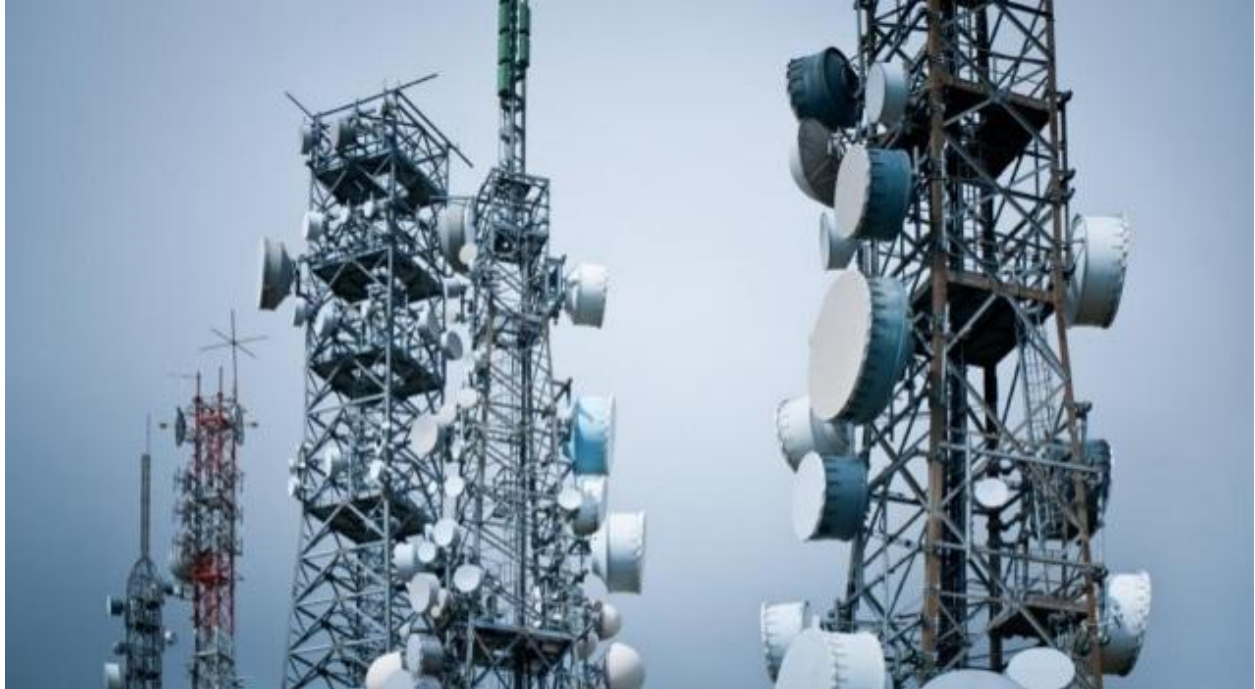
Obr. 1 - Base Transceiver Station
